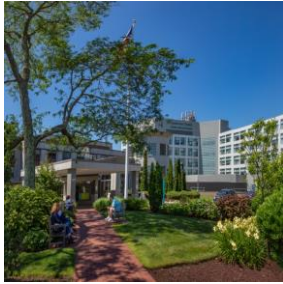
Charlton Memorial Hospital Fall River (1885)
